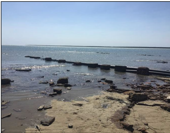
Figure 5: Maningrida Outfall (Power and Water 2016)
