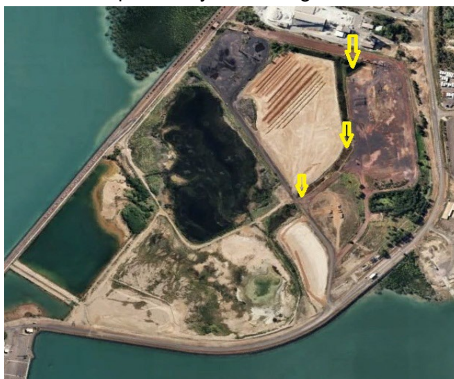
Figure 4 – AGRE water monitoring and treatment locations.
