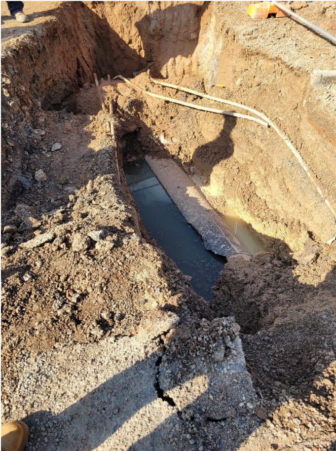
Photo 1 Ruptured Pipe (Photo taken 19/09/2025)
