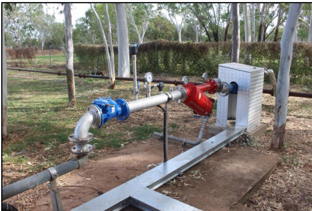
Figure 5. Functioning flow telemetry device at Beswick WwTP
