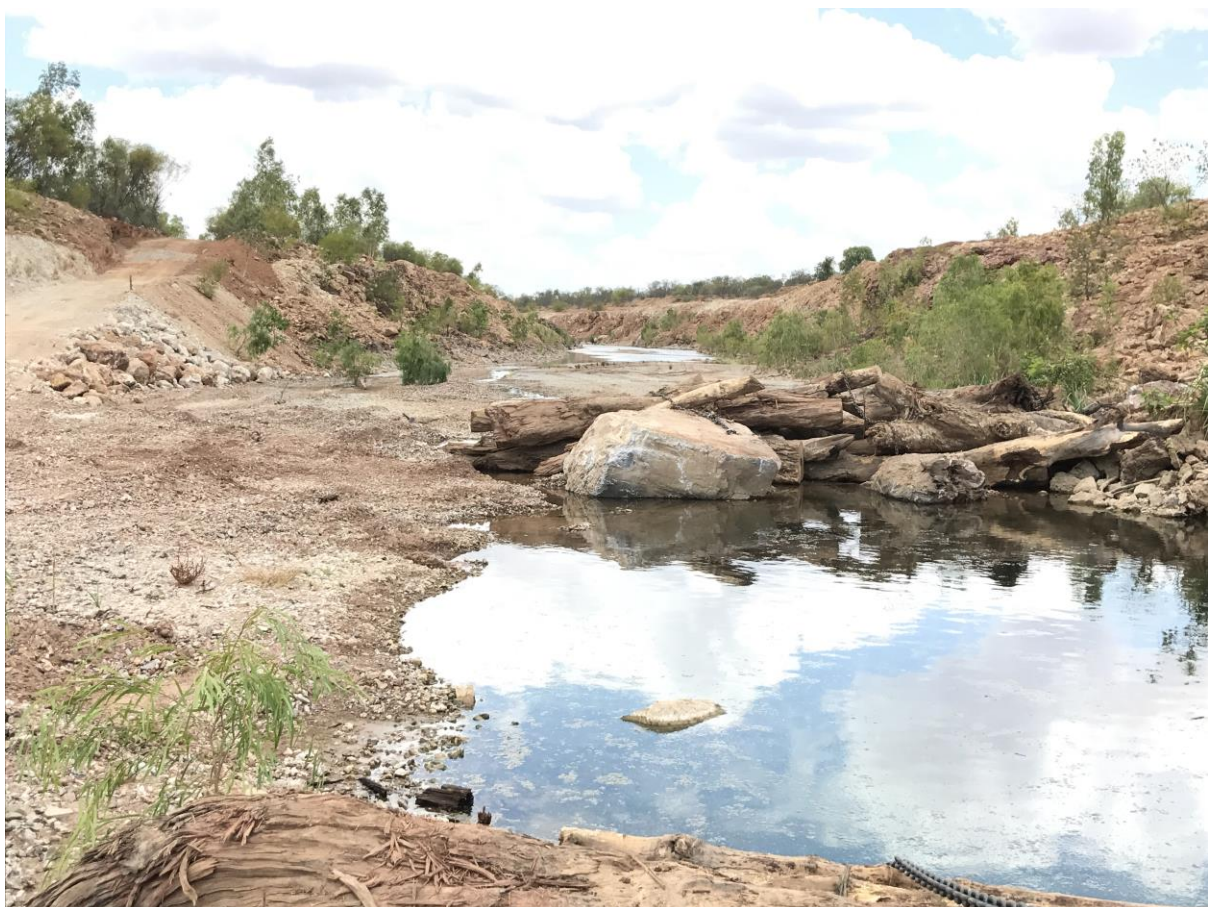
Figure 8-2 McArthur River Diversion Channel
