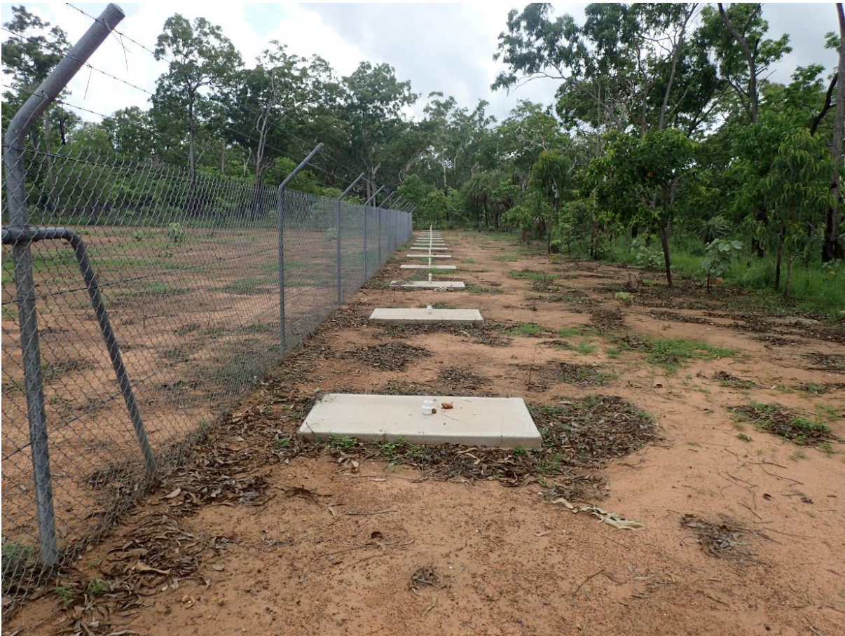
Manthape Wastewater Treatment Plant Discharge Area
