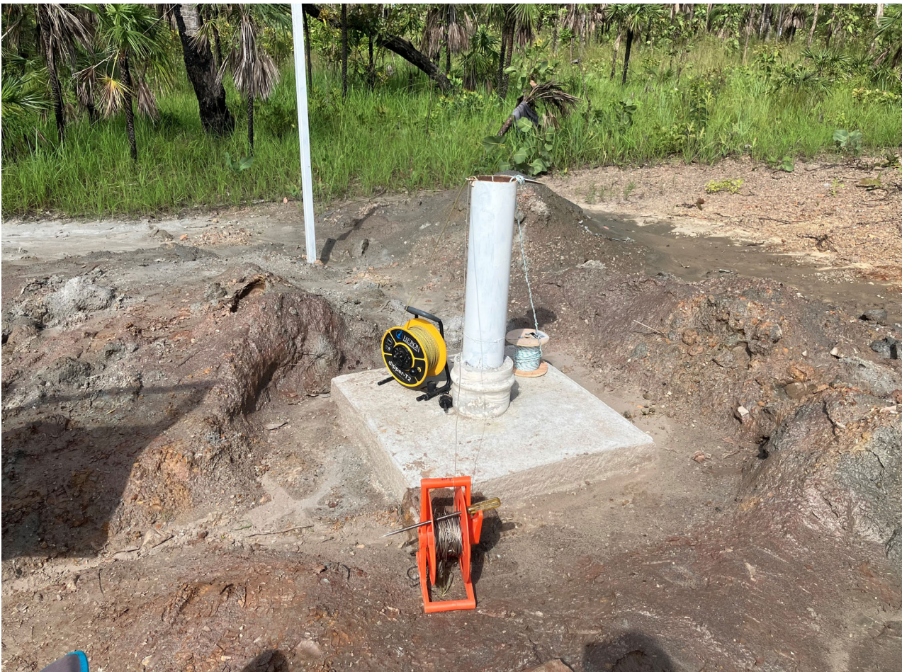
Figure 2-2 Lei Lithium – Final Well Construction during Slug Testing (LG5)
