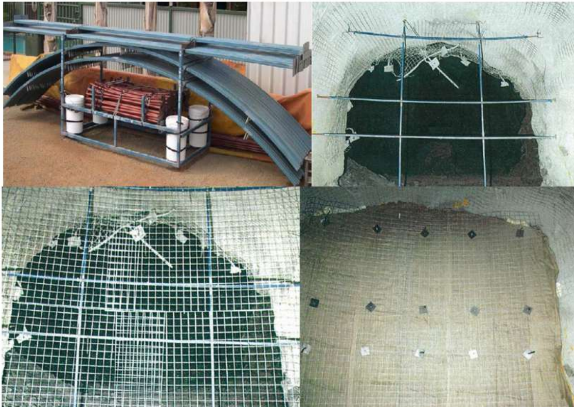
Figure 9.2: Stages of Construction of a Shotcrete Bulkhead
