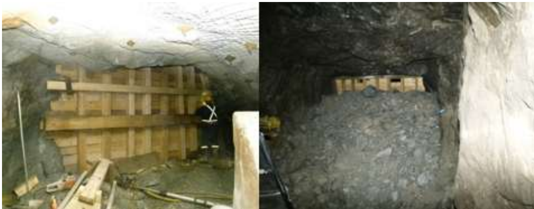
Figure 9.3: Timber Fence (Left) and Waste Rock Fence with Timber Cap (Right)
