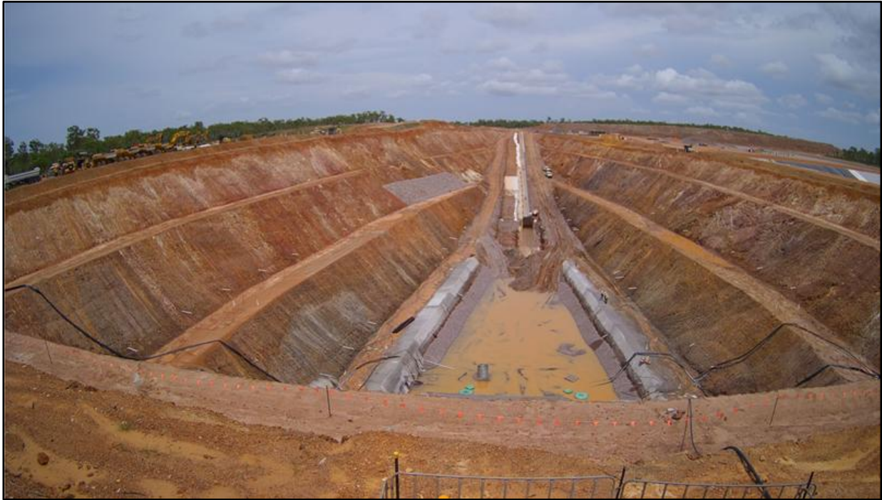
Figure 3-2: View of BP33 Box Cut facing North-West
