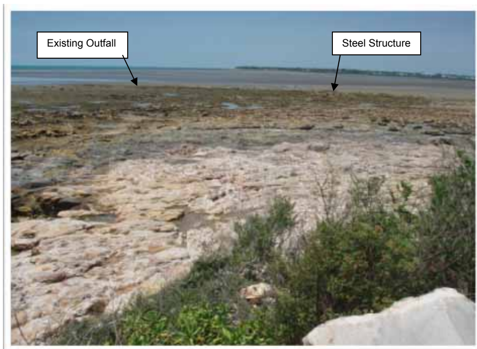
Figure 13 Photograph of the existing East Point outfall and an unidentified steel structure within the intertidal area.
