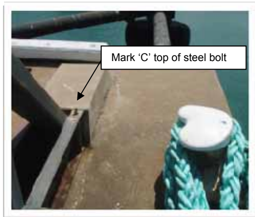
Figure 4 Benchmark on Fort Hill Wharf. (Elevation = 5.892mAHD)
