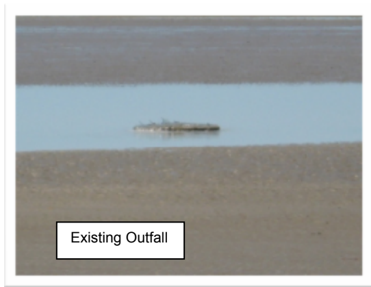
Figure 14 Photograph of the existing East Point outfall
