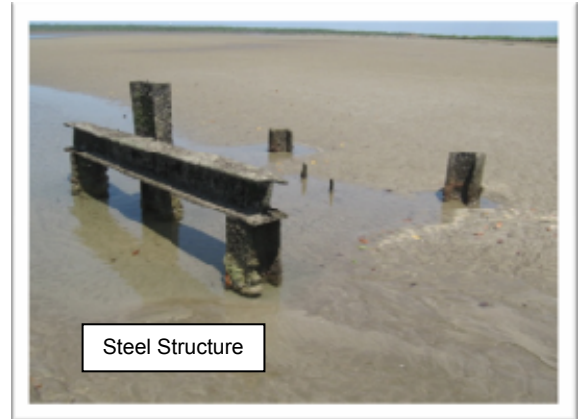
Figure 15 Photograph of the unidentified steel structure
