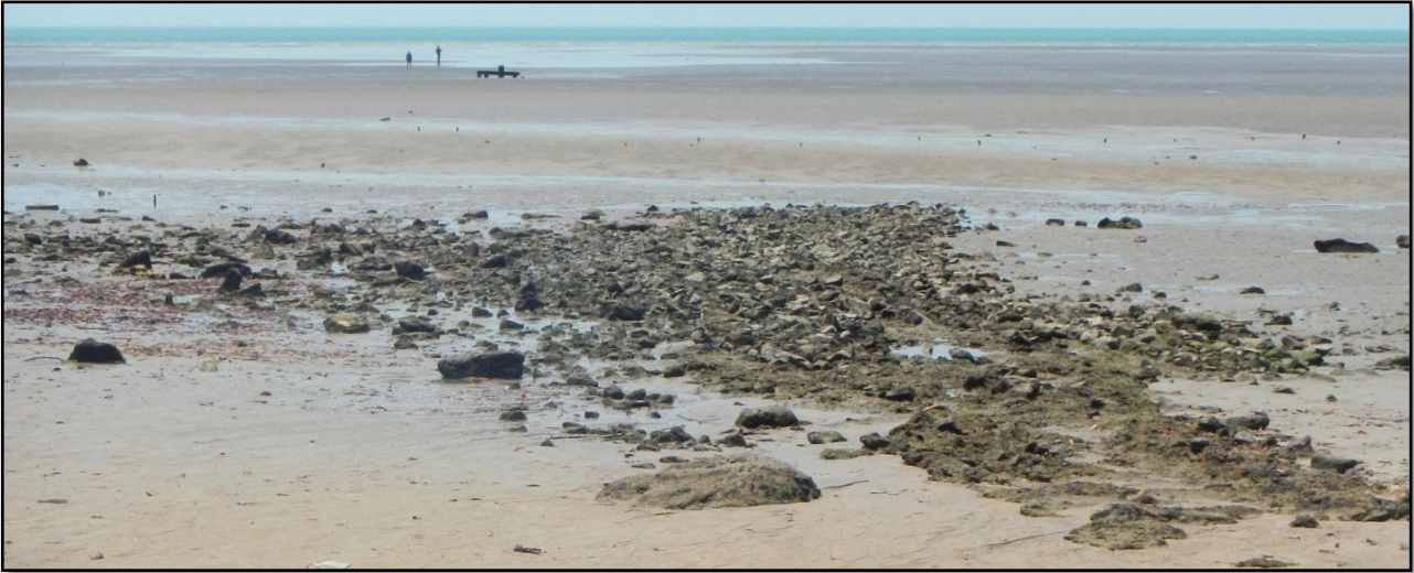
Plate 1-1 Existing East Point Outfall Discharge Point
