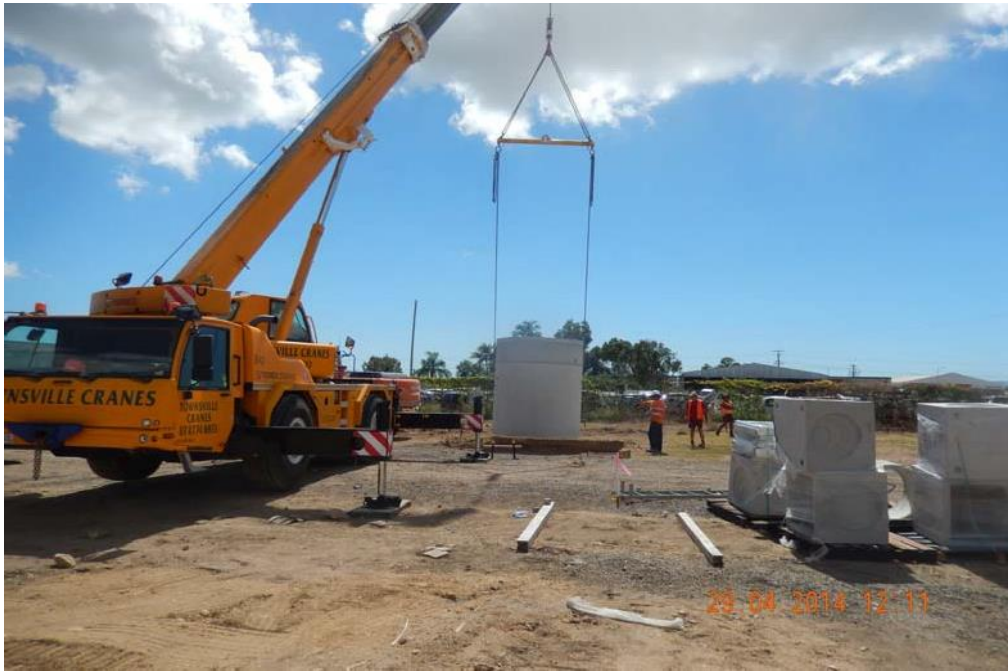
Plate 2 – Installation of a 10,000 litre “Blind Sump”
