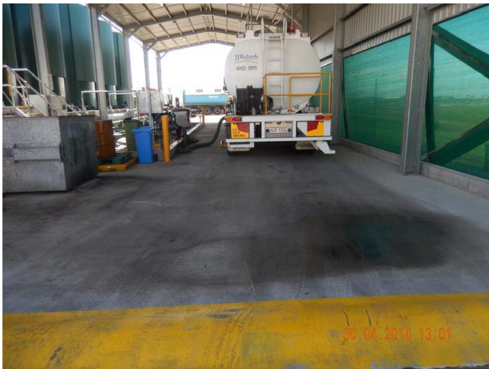
Plate 3 – Truck In Unloading Area
