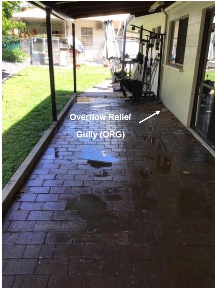
Appendix B – Photographs of the spill site, post clean up.
