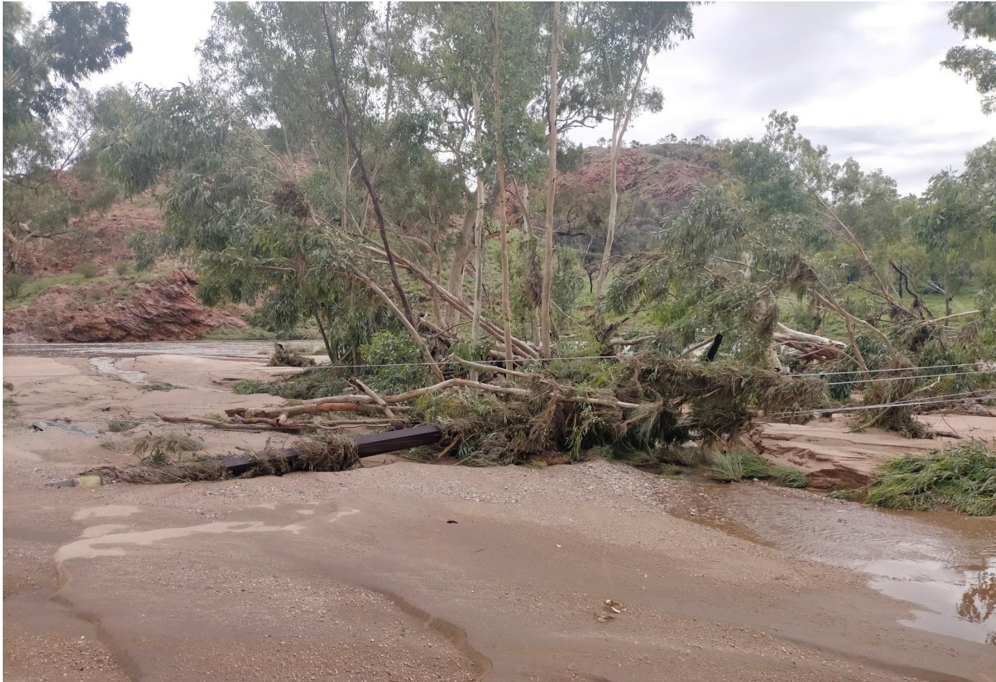
Figure 1: Jay Creek - Potential Receiving Environment (and downed pole)
