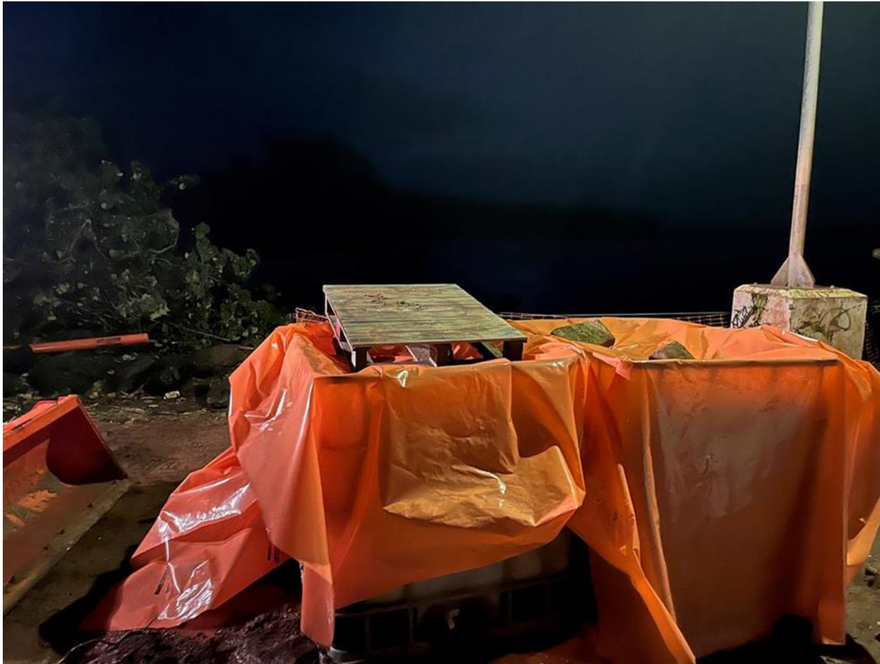
Figure 4. The contaminated soil that was transferred to IBCs and covered with plastic, in preparation for transport back to Darwin.
