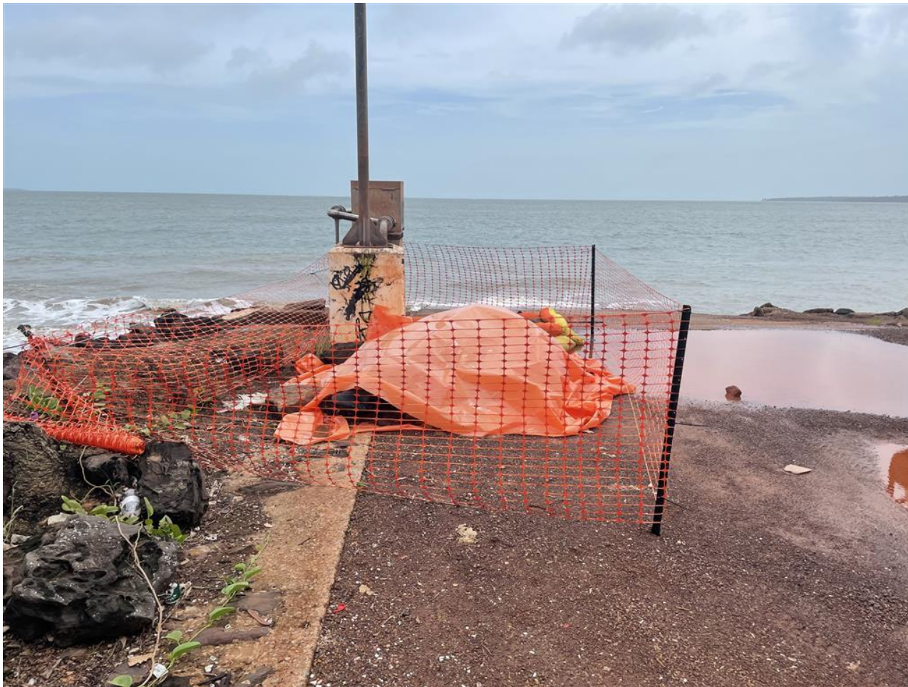
Figure 2. Initial excavation's contaminated soil covered with plastic, with spill booms just visible behind the mound.
