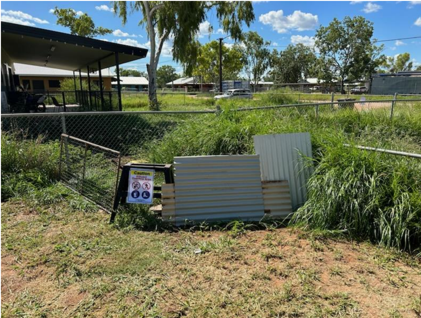
Figure 1 - Spill source, barricaded as best as possible with materials available.
