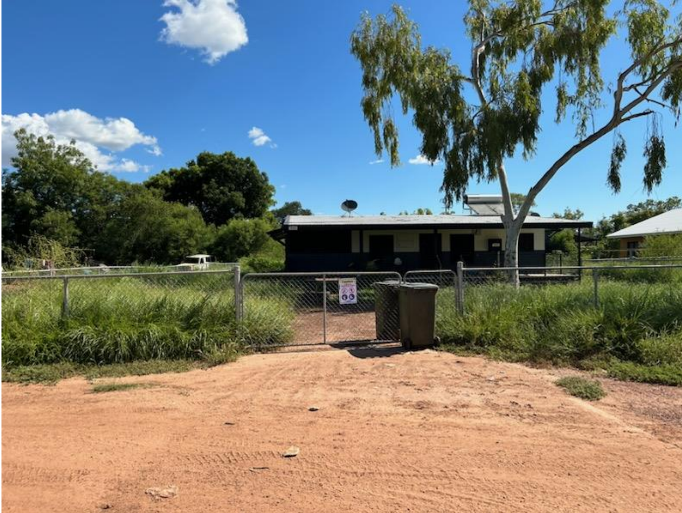
Figure 2 - Warning signage on display at affected property boundary entry point.
