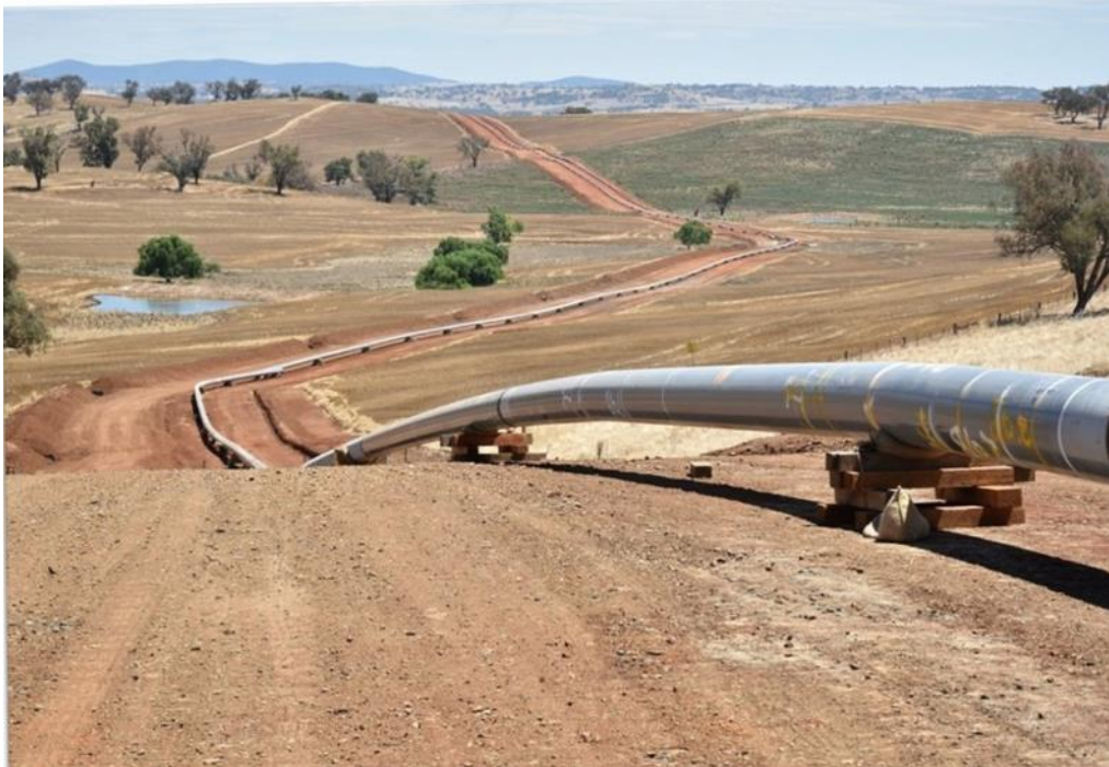
Figure 3.15 ROW during construction
