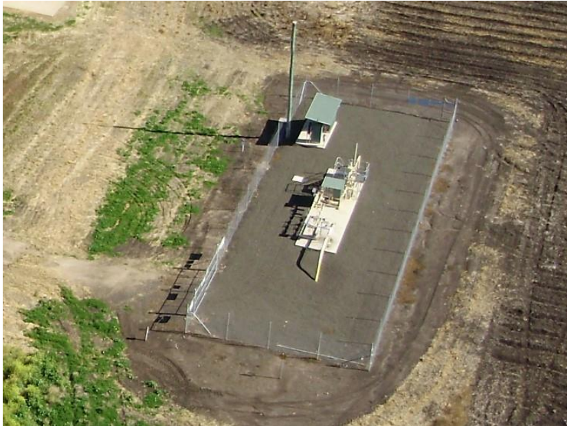
Figure 3.5 General photo showing an above ground facility
