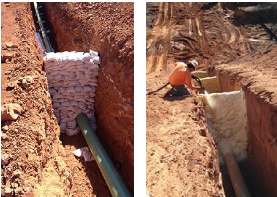
Figure 3.14 Example of trench breakers
