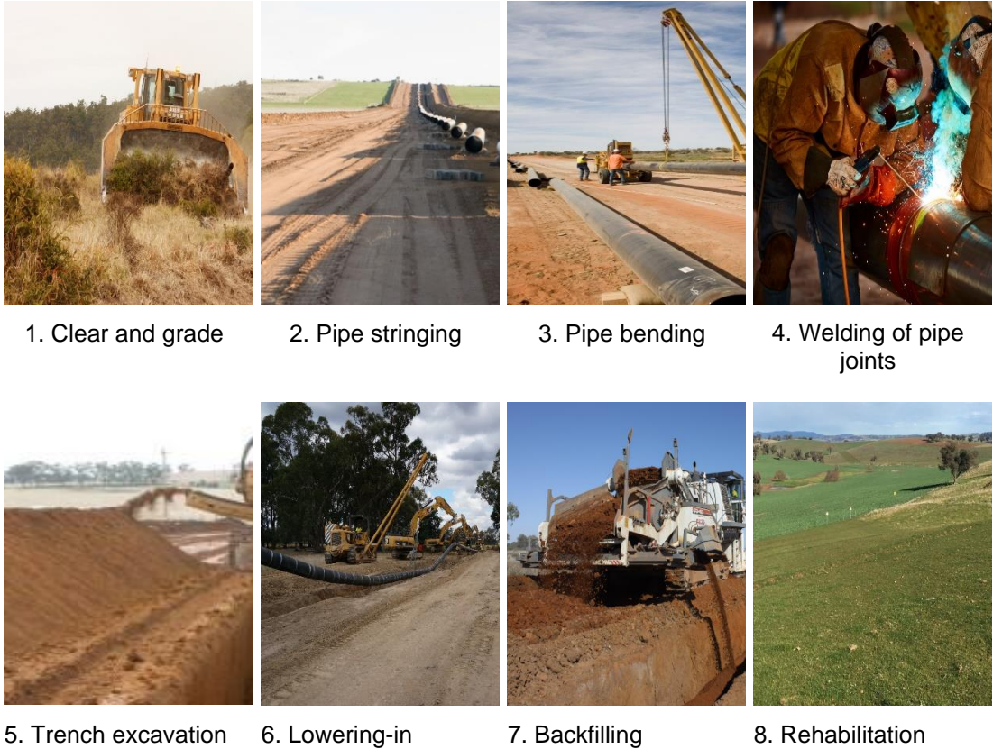
Figure 3.11 Pipeline construction sequence
