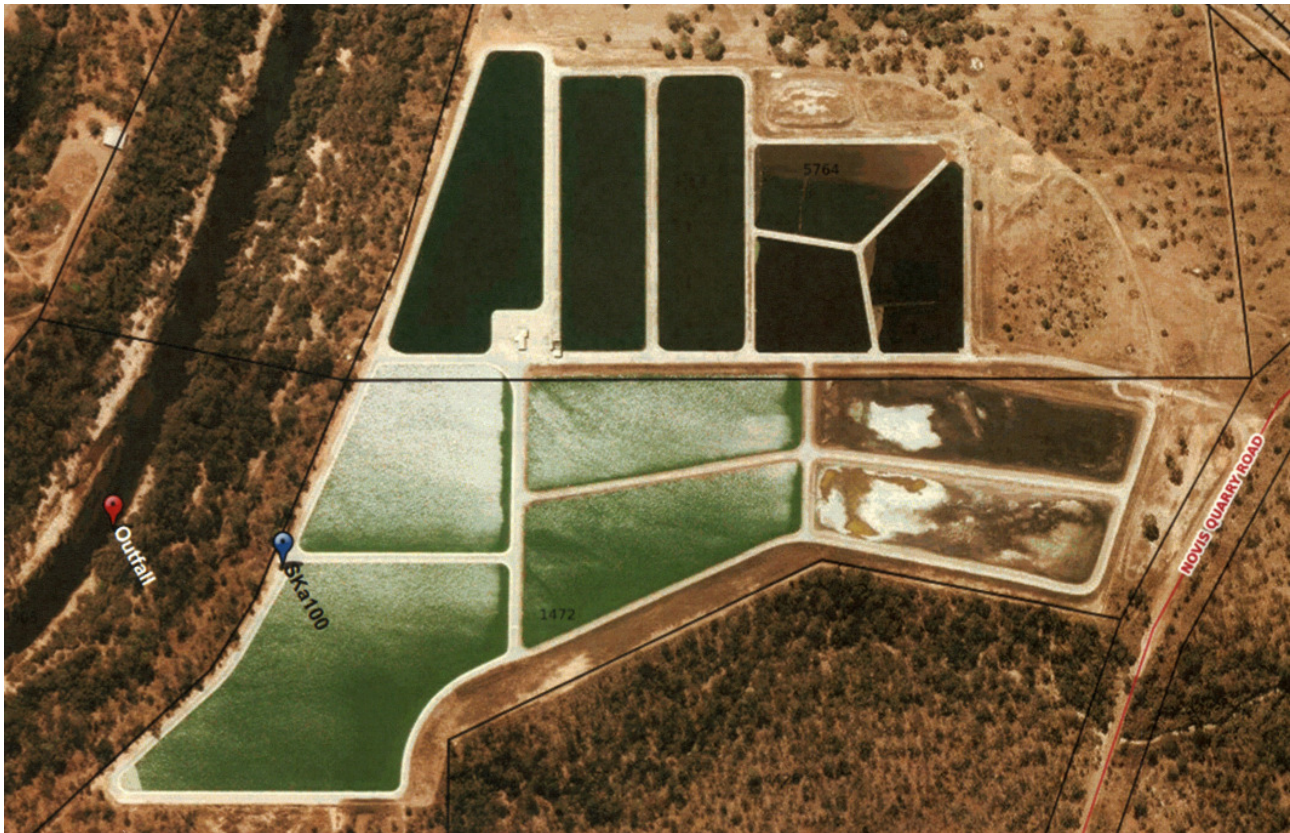
Figure 3: SKa100 - authorised monitoring location/sampling point.
