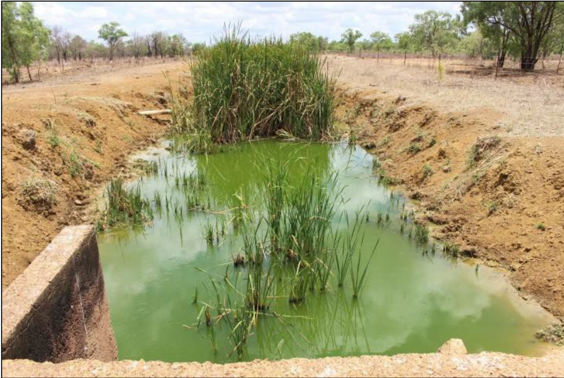
Figure 6. Effluent discharge point to open unlined drain (PWC 2017)
