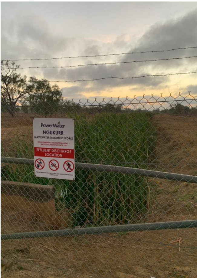
Figure 7. Effluent discharge point to open unlined drain in 2021 (PWC 2021)
