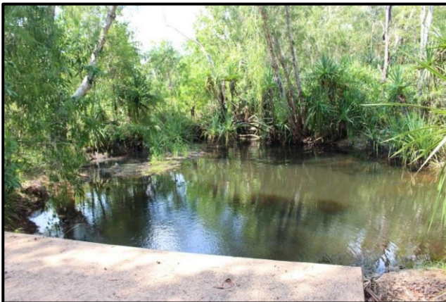
Figure 5. Manton River causeway located near WwTP (PWC 2025)
