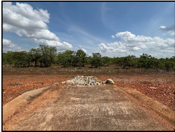
Figure 8. Rock Spillway located on pond 4 (PWC 2025)
