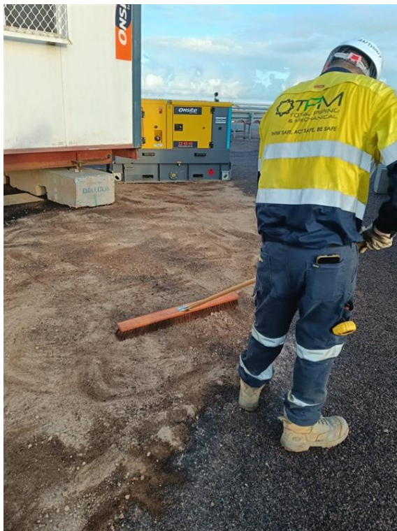
Cleaning In Progress 3
