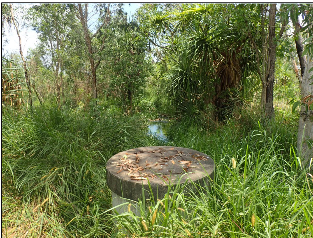
Figure 5: Wadeye outfall receiving environment (13 December 2016)
