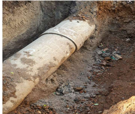
Figure 4: Excavate around and beside pipe
