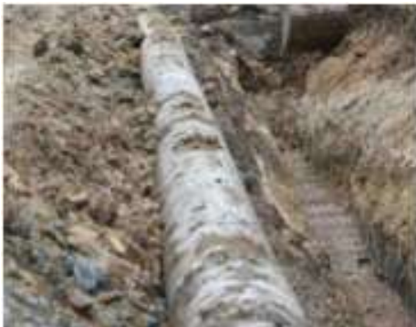
Figure 4: Excavate around and beside pipe
