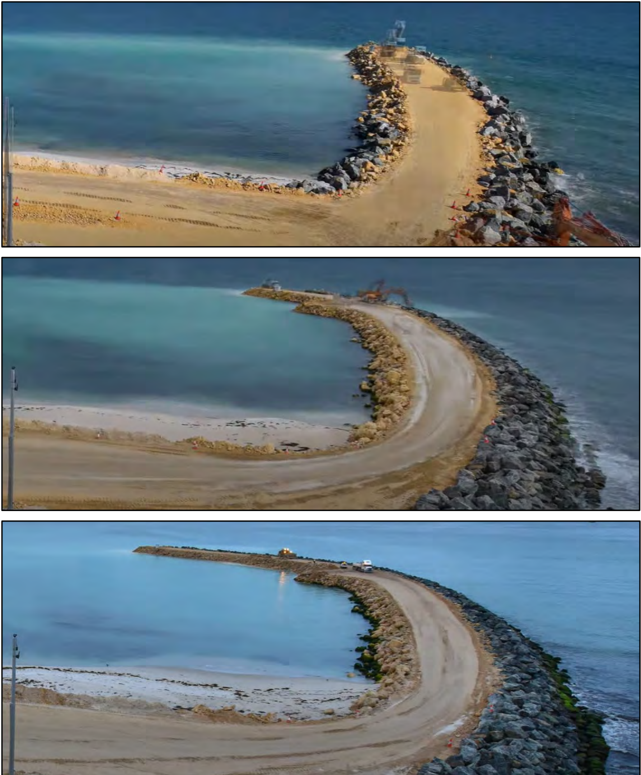
Figure 2-5 Example of staged breakwater construction (Ocean Reef Marina – DevelopmentWA, 2021)
