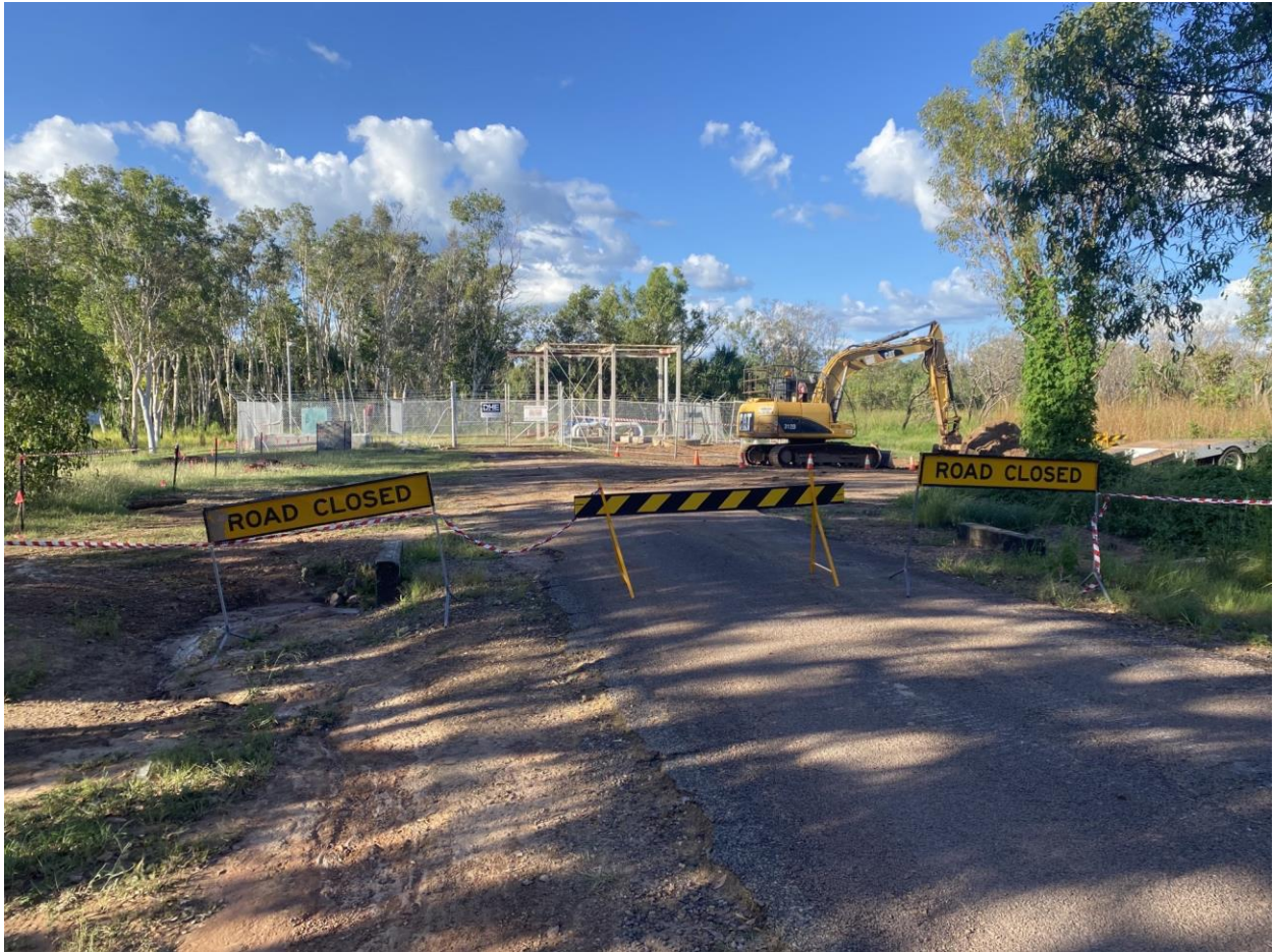
Figure 4: Site Secured with temporary Fencing
