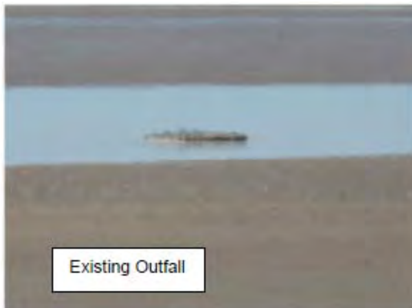
Plate 1-1 East Point Outfall on low tide
