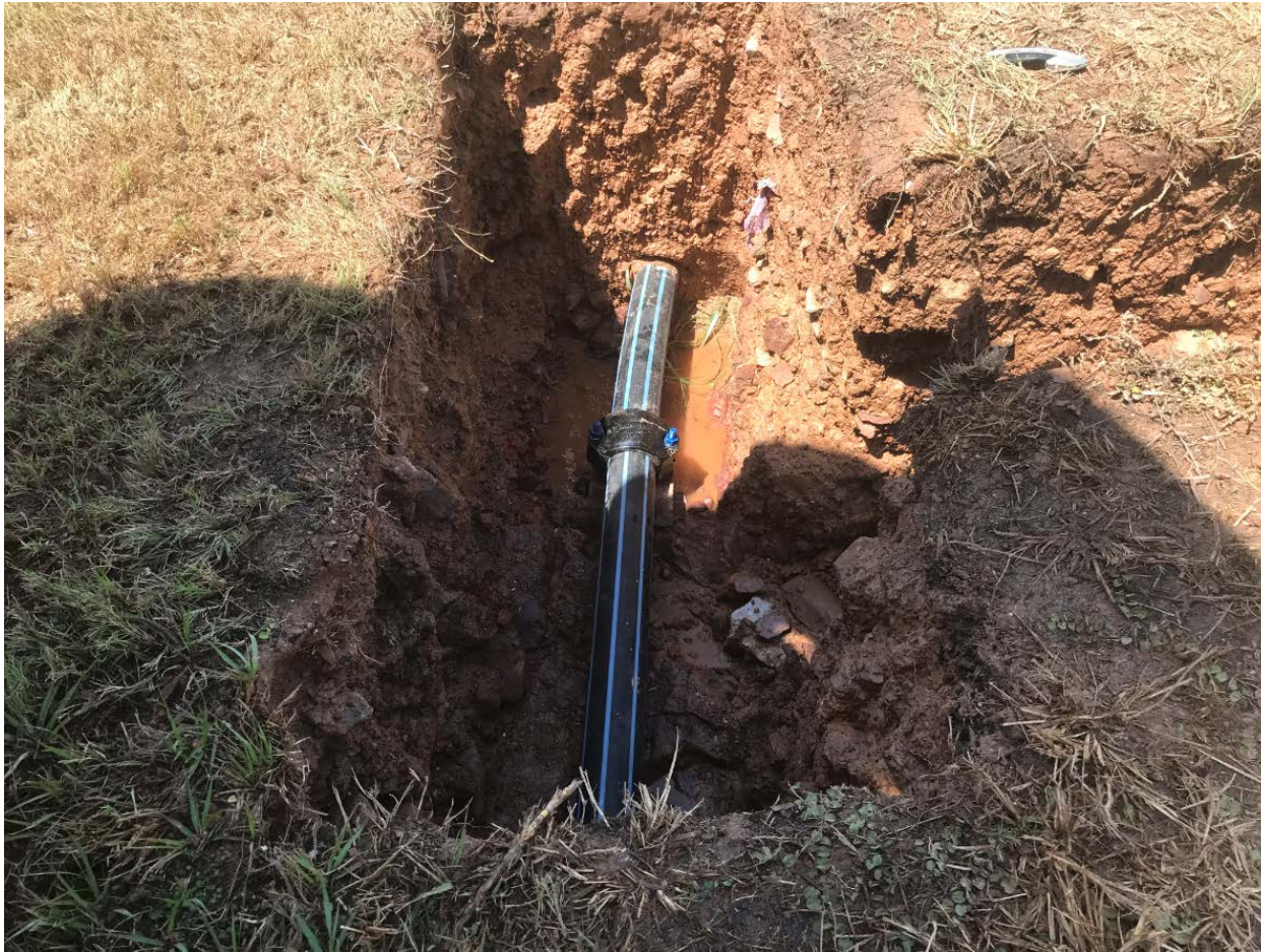
Photo 1 – Repaired sewer rising main
