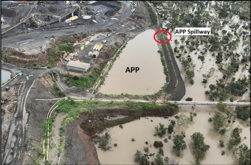
Figure 4. Location where BC floodwaters inundated the Mill Pond.
