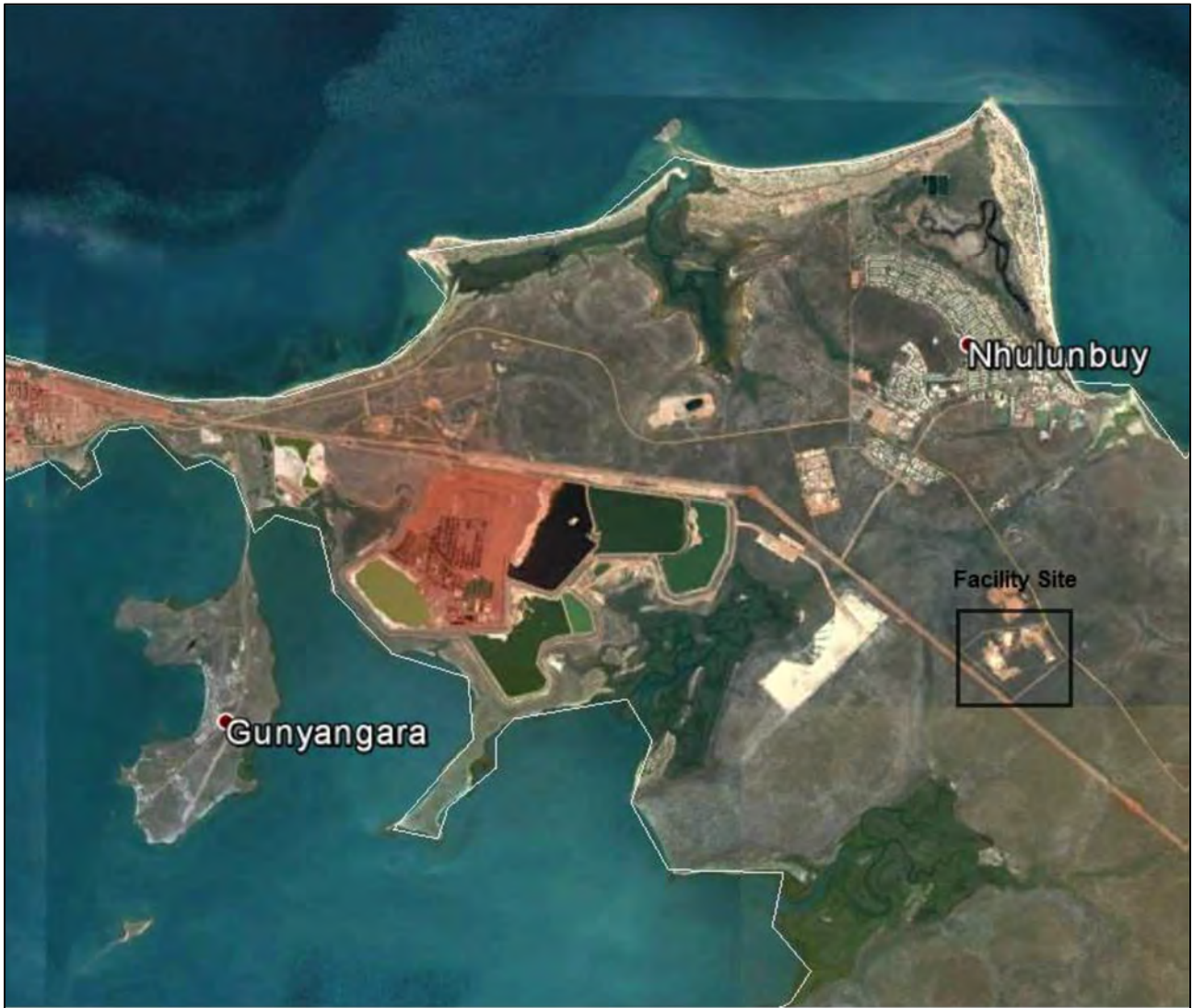
Figure 1. Locality plan of Gove Peninsula Waste Management Facility. Image taken from the WGMP.
