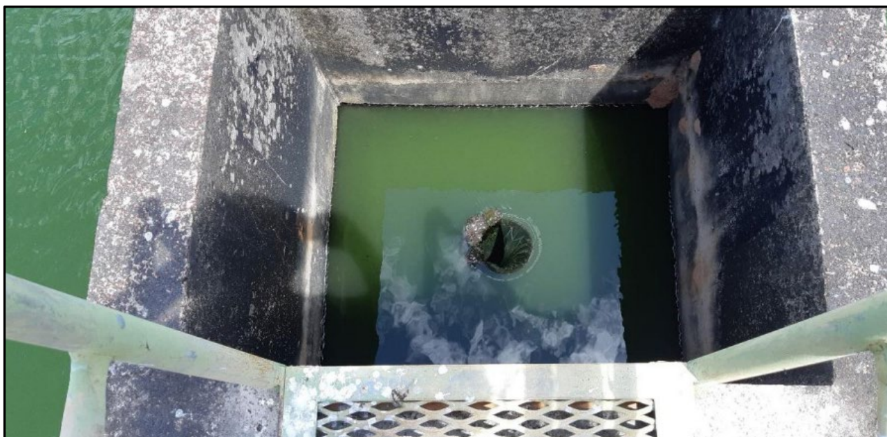
Figure 5: Image of concrete effluent discharge pit (PWC 2021b)
