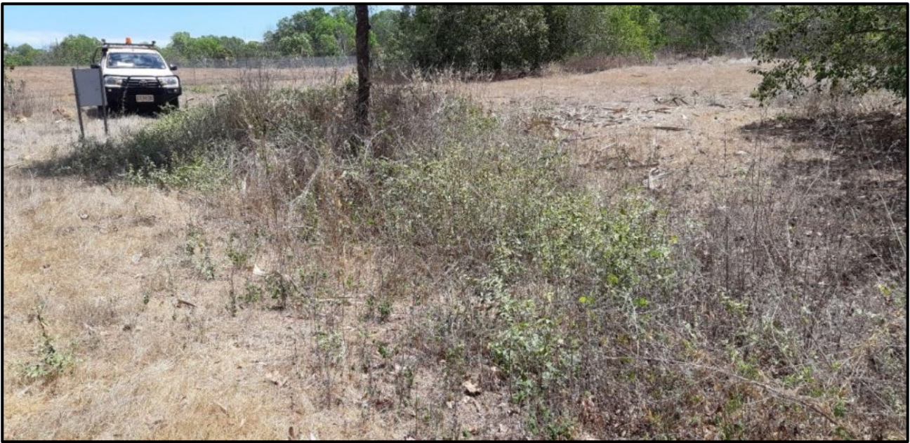
Figure 7: Culvert located nearby the WwTP where discharge pipe occurs (PWC 2021b)
