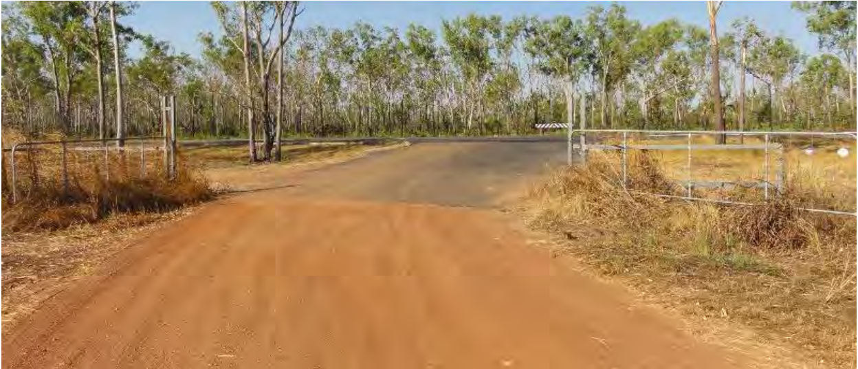
Photograph 2 – Access road approach to Stuart Highway – bend restricts vision to the intersection to approximately 50 m.
