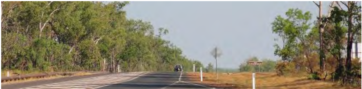
Photograph 3 – Looking south from the abattoir access at Stuart Highway
