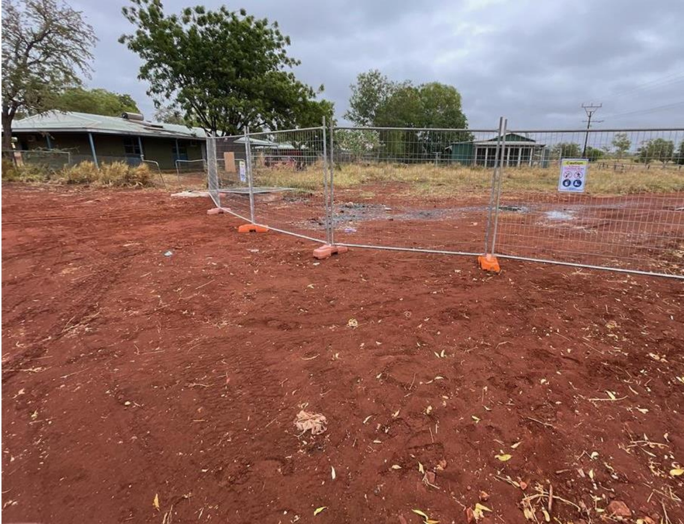
Figure 2 – Showing secure pedestrian fencing erected around the spill, now with appropriate warning signage.
