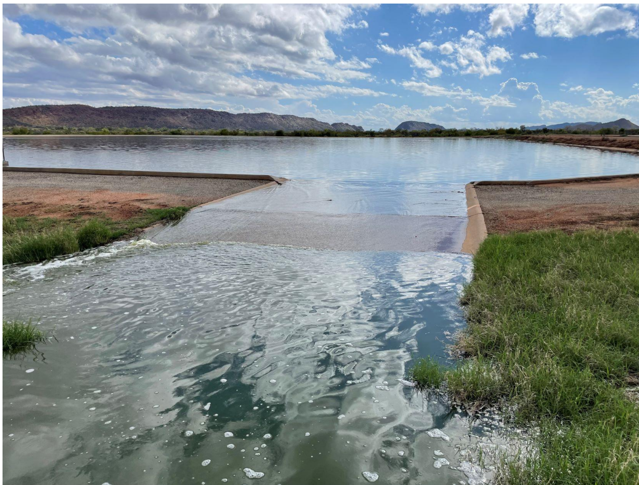
Image 1: Discharge from Pond C3. Historical image used.
