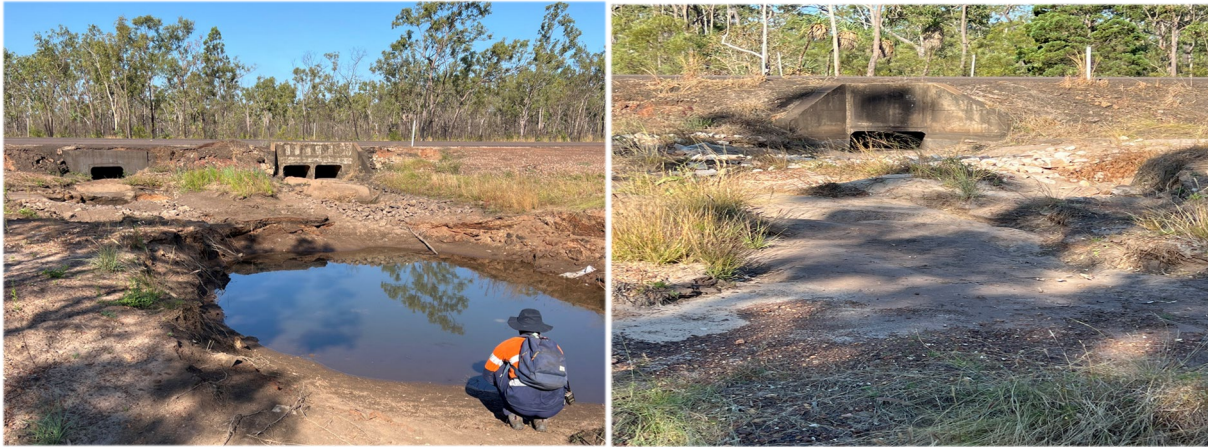
Figure 15 Largely dry drainage lines leading to culverts under Rowell Highway observed during August 2024 surveys
