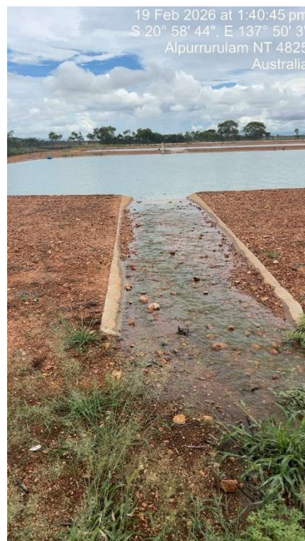
Figure 2 – Emergency overflow channel
