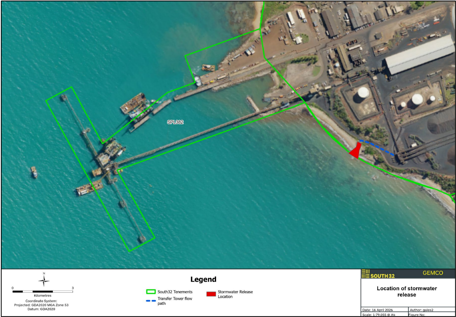
Figure 1: Location of stormwater release.
