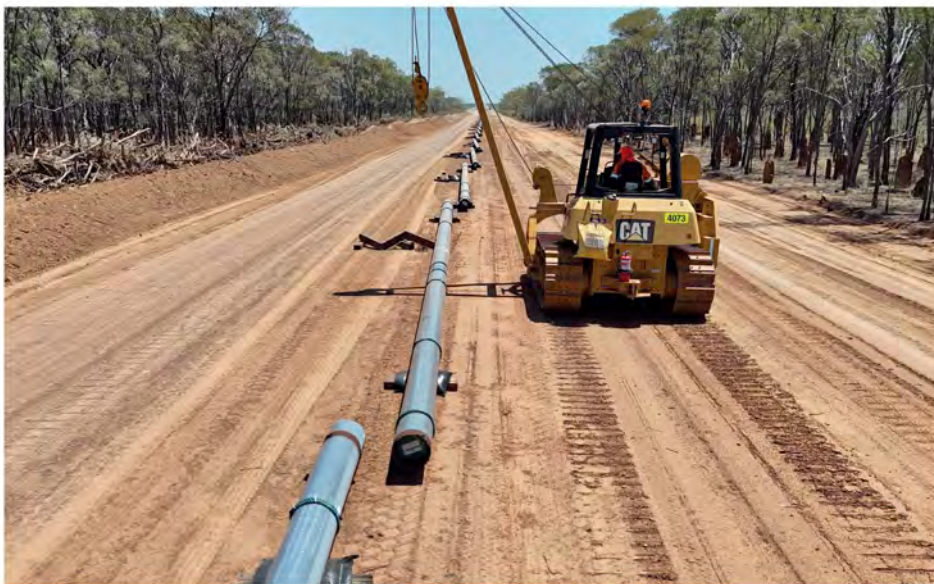
The pipes are lined up on the ground.
