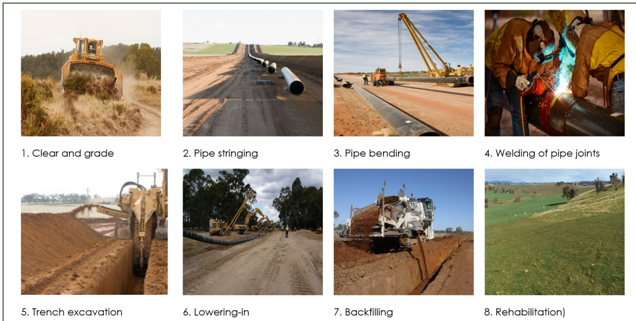
Figure 2 Pipeline Construction Sequence
