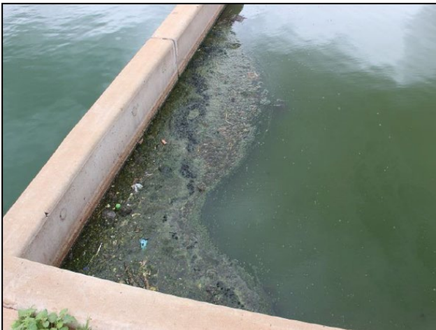
Figure 8: Minimal surface scum observed at ponds (PWC 2018)
