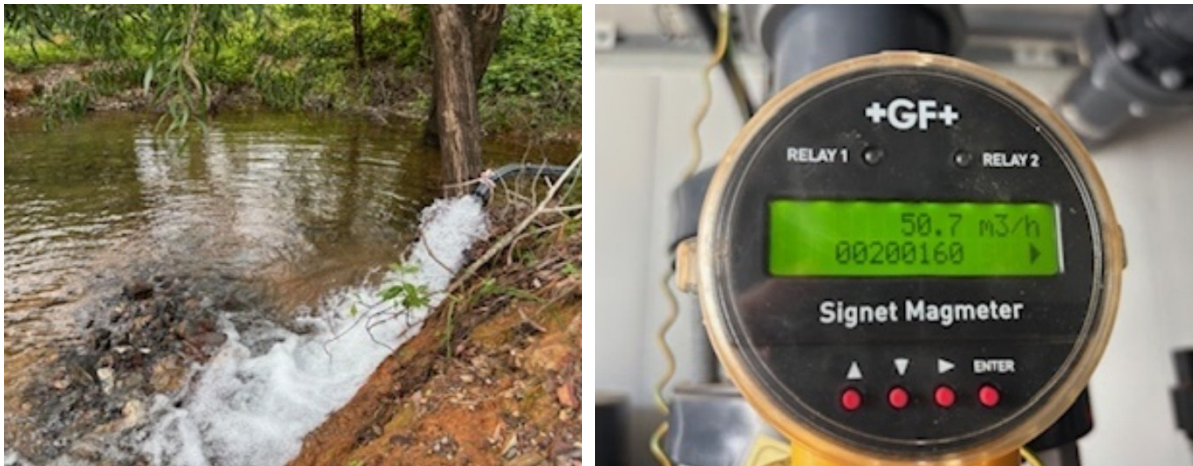
Photo 4-1 Authorised Discharge Point pond and flow meter
