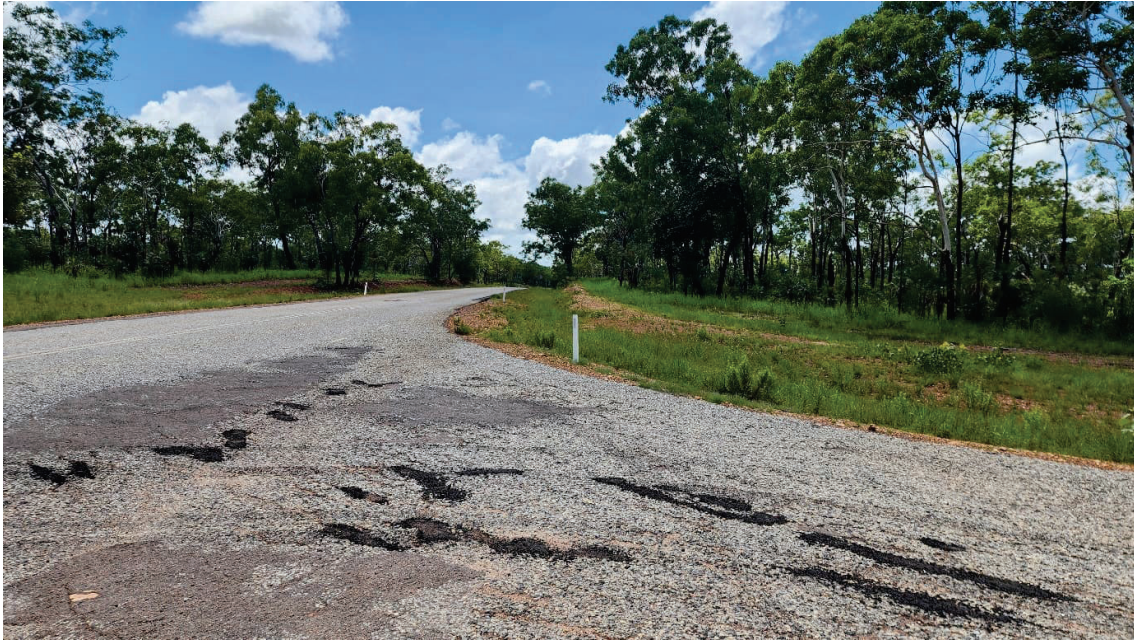
Figure 10 Sight distance restricted by crest at BP33 mine access
