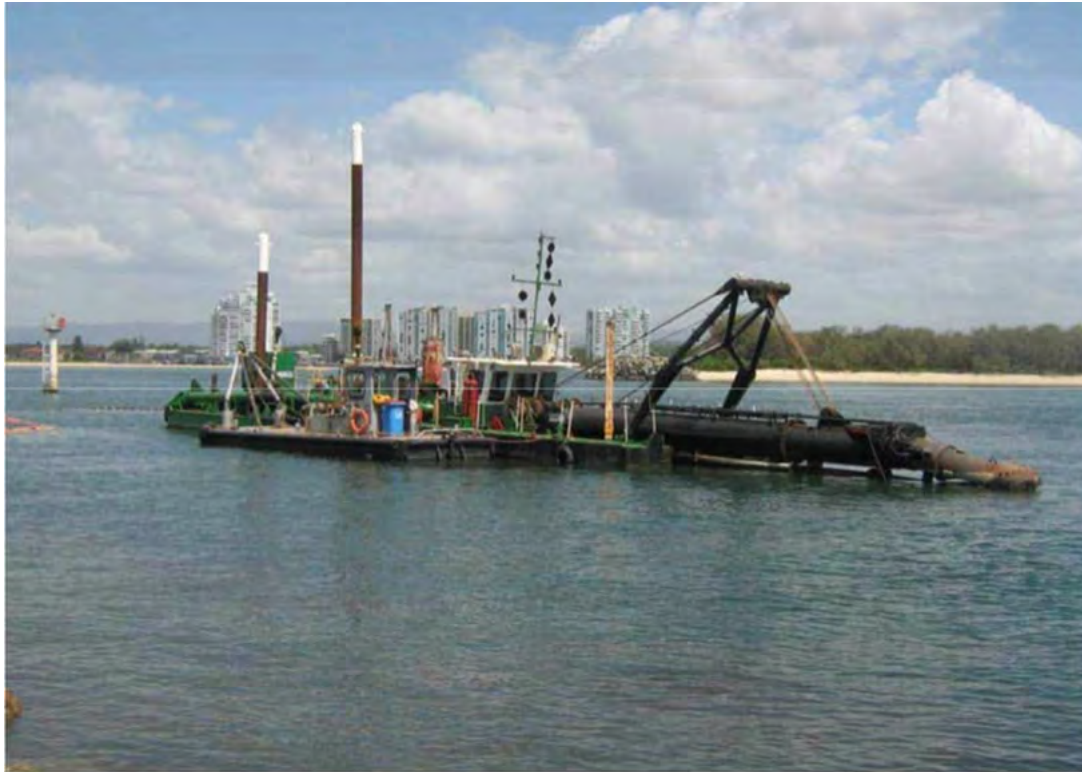
Figure 4-3: CSD Everglade (Hall Contracting) (source: Hatch 2024)
