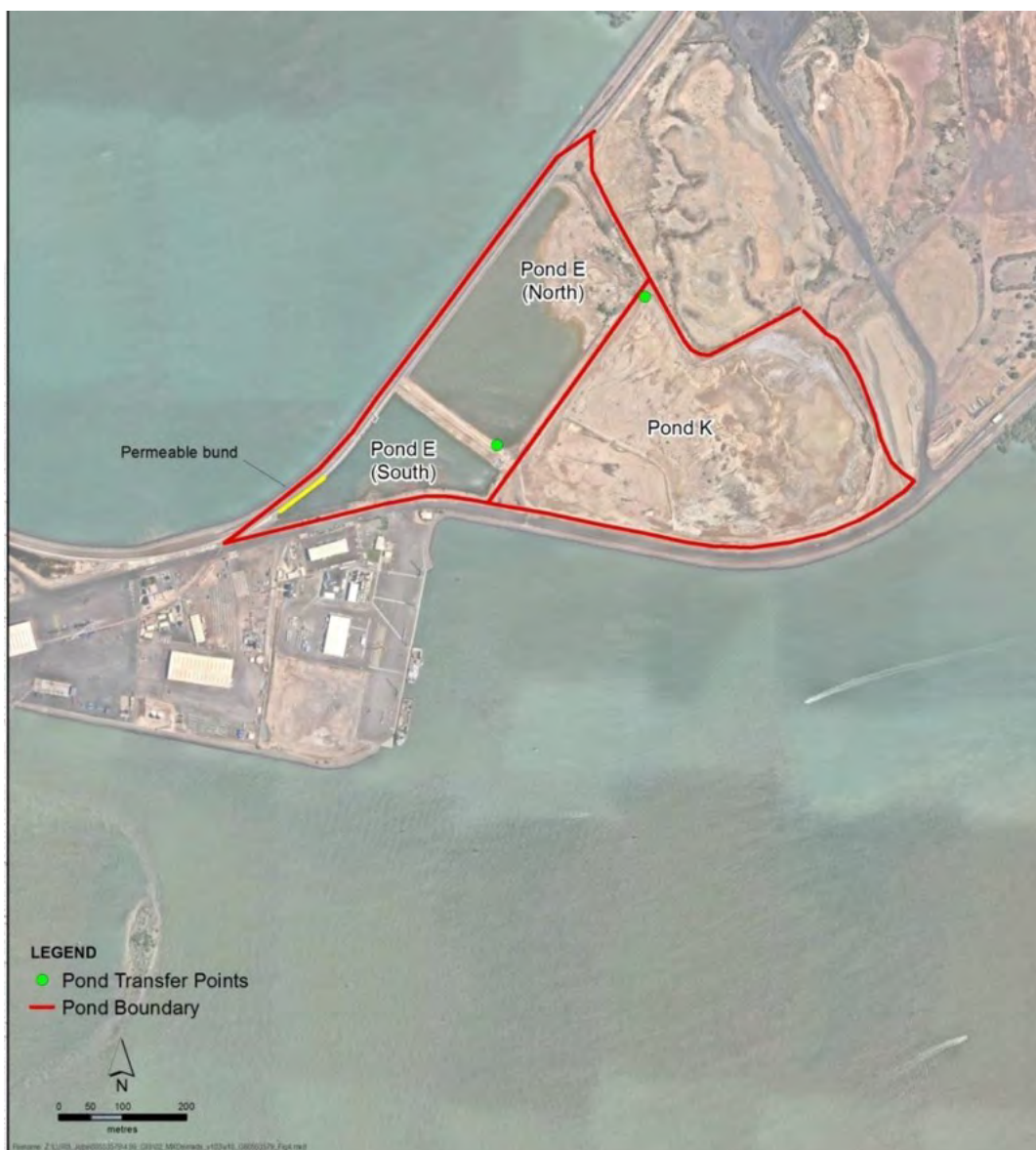
Figure 4-7: East Arm Wharf Pond system
