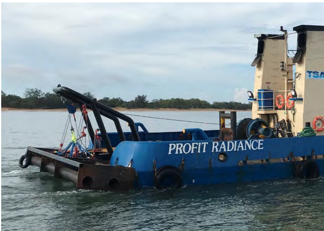
Figure 4-2: Close up of the type of bed levelling equipment (example only) to be used for the works.
