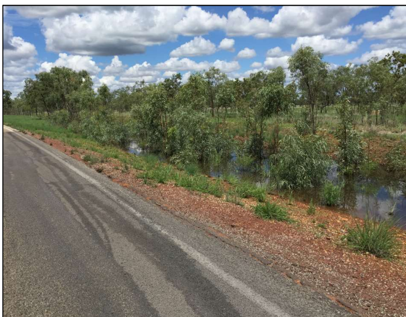
Figure 4 – Roadside runoff drain.
