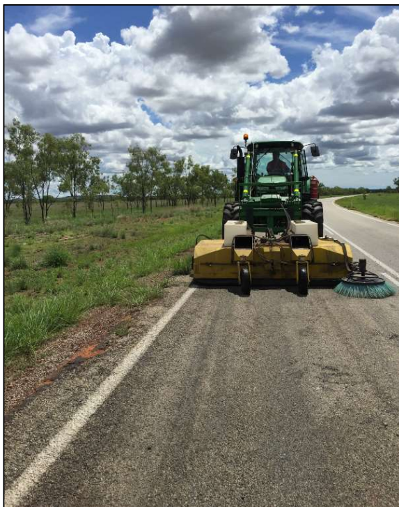
Figure 3 – Concentrate spill site during the clean-up.
