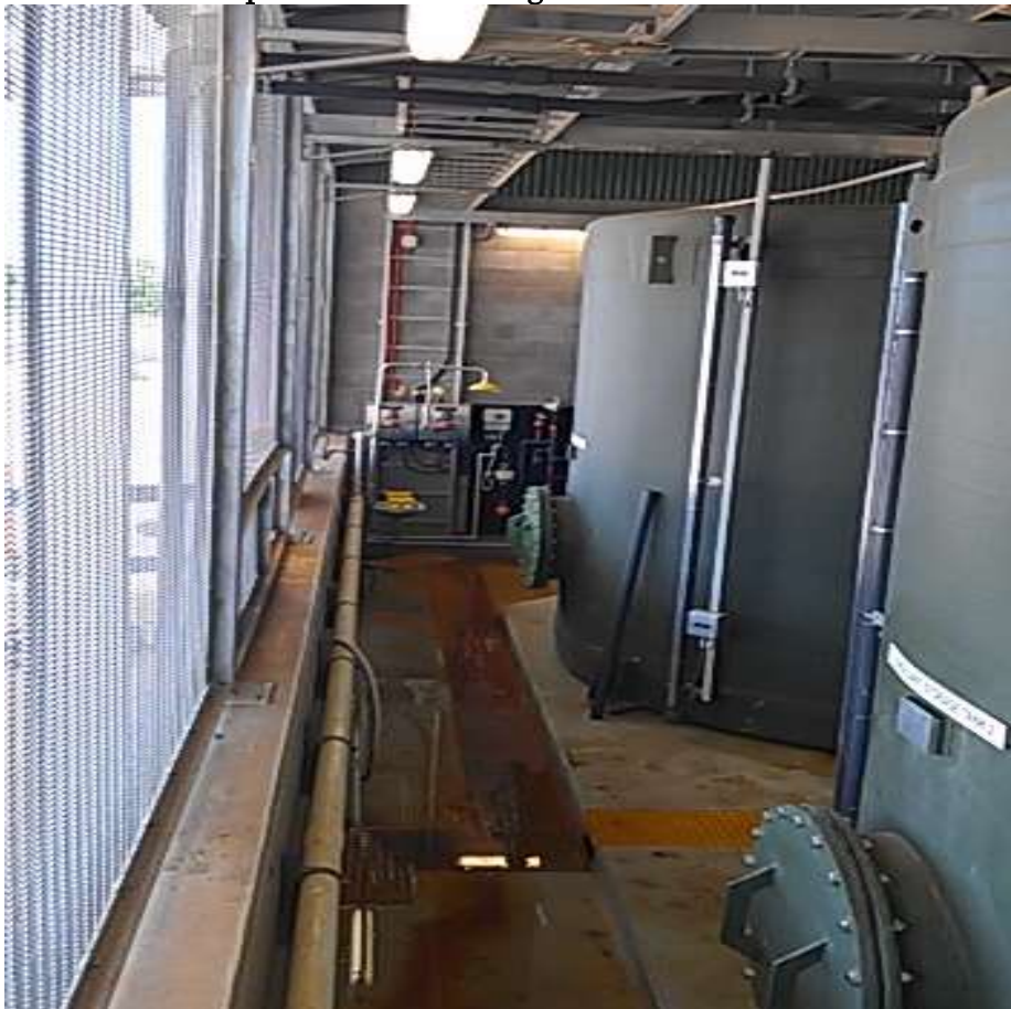
View of outside Coagulant tank room. Ferric Sulphate solution tanks and bund
