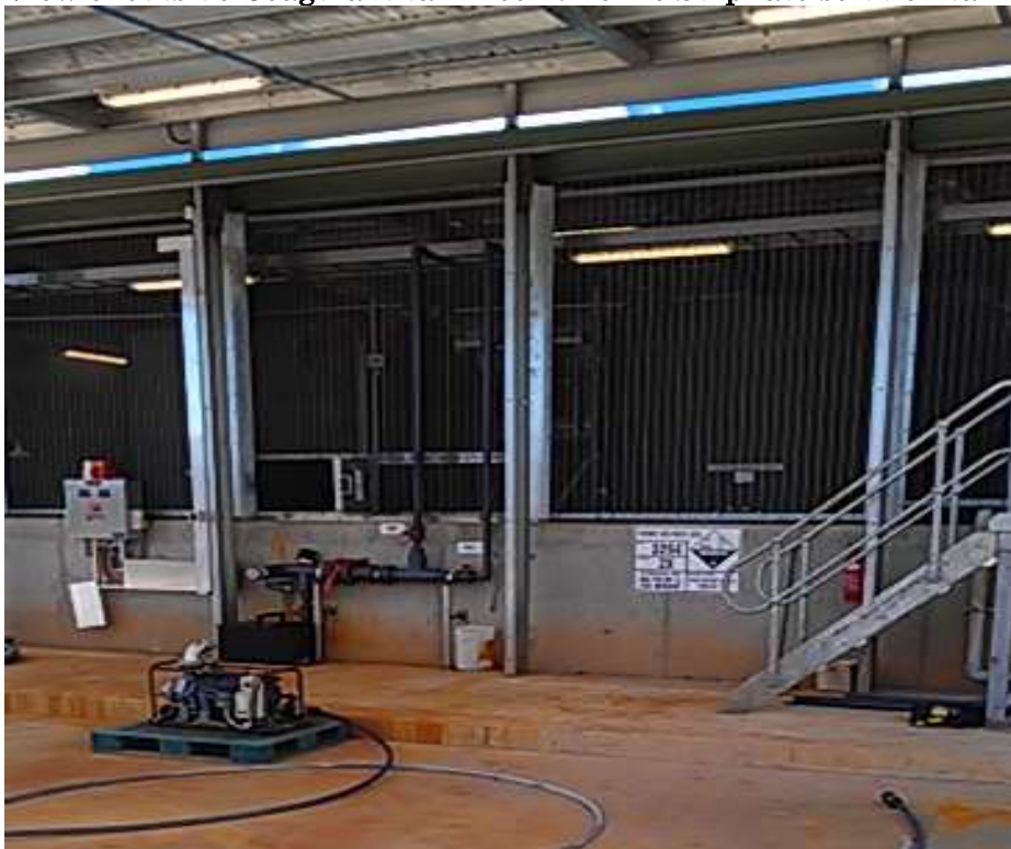
View of outside Coagulant tank room. Ferric Sulphate solution tanks and bund
