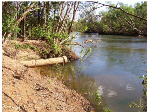
Figure 3 Discharge pipe from KWwTP to Katherine River (PWC 2019)
