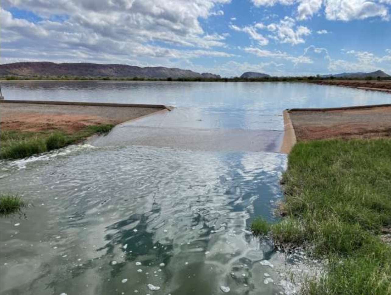
Photo 1: (Point 1 as per Section (b)): Discharge from Pond C3 Taken 16:04hr 10/11/2021
