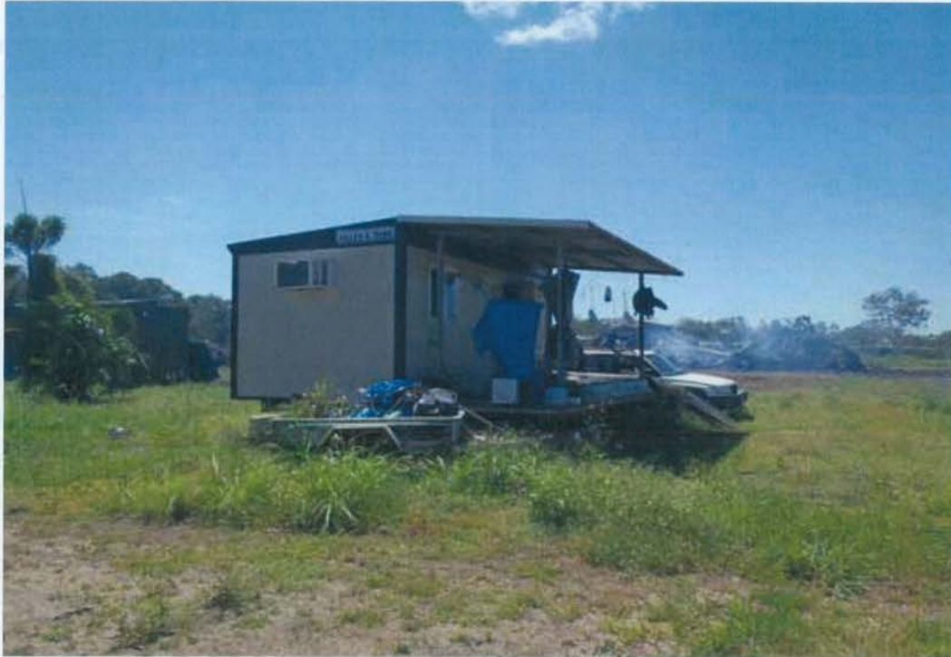
Photo 11: View of temporary structure, from near TP6 and facing east
