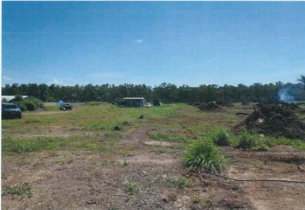
Photo 3: View of site, looking north from southeast site corner
