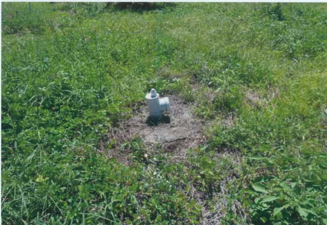
Photo 16: View of concrete cover to septic system
