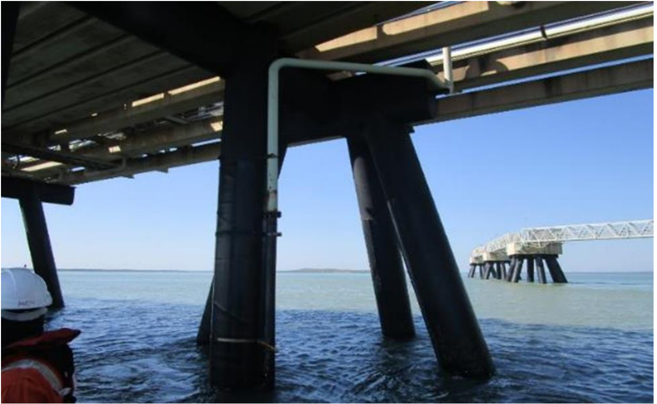
Figure 3-2: DLNG jetty outfall pipe (secured to pylon)
