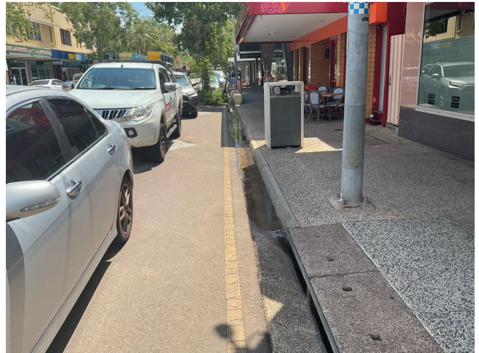
Figure 4 – Final discharge point (stormwater drain)
