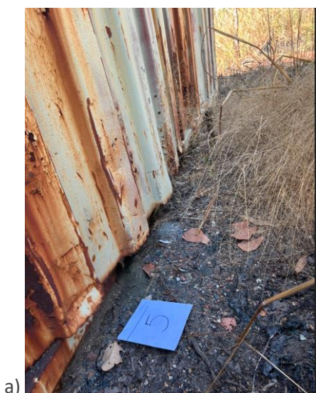
Figure 47a. Buckling of the side wall on container 5, integrity of the container has been breached along the bottom. b) and side c) Close up of rust along the wall looking towards the end of the container.
