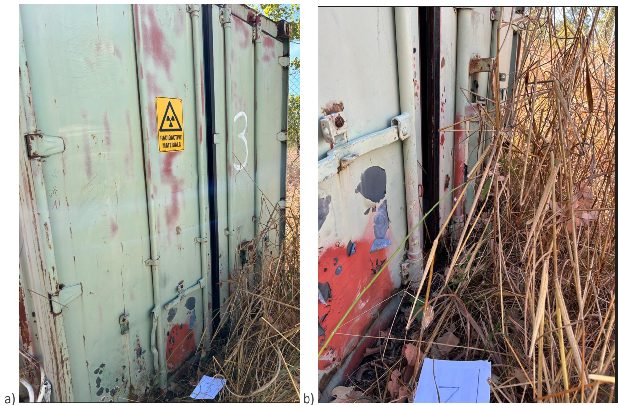
Figure 32a. Photo showing shipping container #3 door. The radioactive materials labels can be seen affixed to the door. The door has not been chained or locked due to difficulties doing this (likely due to door mechanisms seizing due to rust and environmental conditions). b) There is a gap where the 2 doors meet of about 5cm or less.
