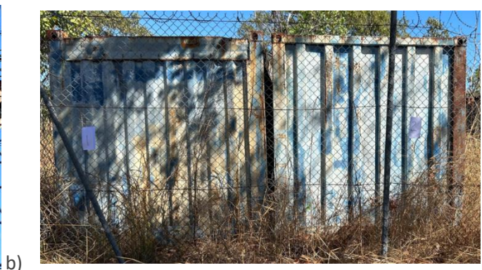
Figure 26b. Photo attempting to show the slight lean of shipping container #1, at the top of the fence line the shipping container is much closer to it than it was at the bottom. b) Photo showing positioning of shipping containers #1 and #2 next to each other.
