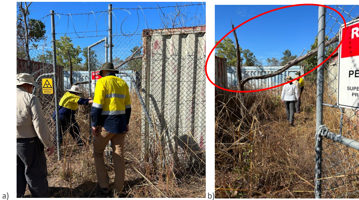
Figure 20a. Grass growth inside the fenced enclosure being pushed out of the way when the gate was opened. A fallen tree growing inside the enclosure can be seen in the background. b) close up of the central fallen tree which has a branch fallen on container #4. Movement through the enclosure does a great job of quickly flattening the overgrown grass.
