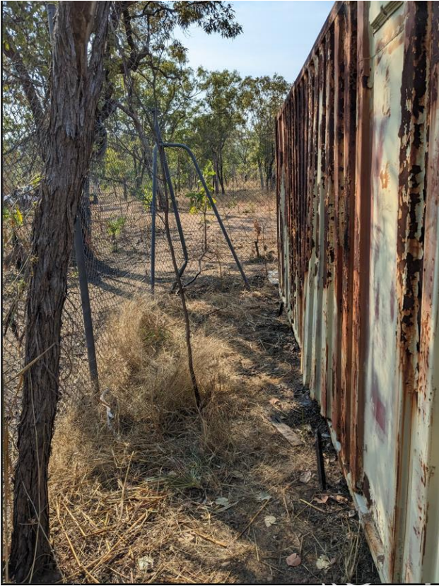
Figure 46. Photo of long side of shipping container #5.
