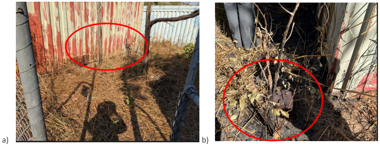
Figure 21a. Debris inside the enclosure - old broken chairs inside the enclosure near shipping container #3 and old oil can near door of container #4. b) The ground in front of shipping container #4 and #5 appears to have burnt debris in front of it – refer to pictures for shipping container 4 and 5 for close up details
