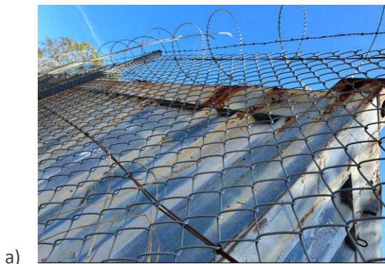
Figure 26b. Photo attempting to show the slight lean of shipping container #1, at the top of the fence line the shipping container is much closer to it than it was at the bottom. b) Photo showing positioning of shipping containers #1 and #2 next to each other.
