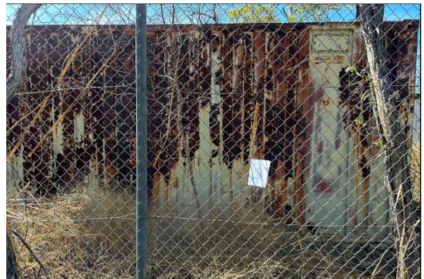
Figure 49a. and b) Photo showing condition of side view of shipping container #5 on the fence side. Rust is clearly visible. The other side of container #5 abuts onto shipping container 4 so no photos of the other long side are possible.
