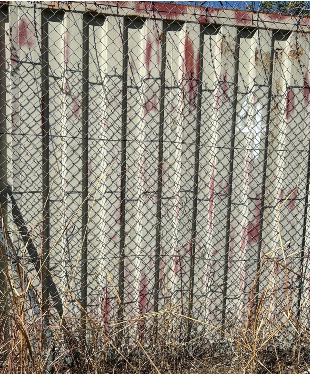
Figure 41. Photo showing condition of end view of shipping container #4
