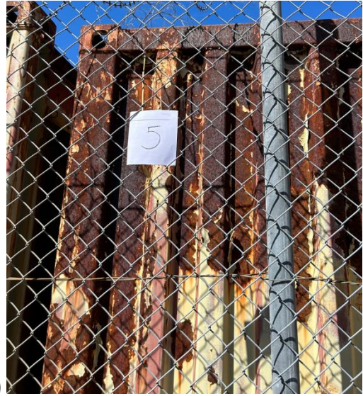
Figure 50a. and b) Close up of the rust on shipping container 5, long fence side, towards the door end, and end side next to shipping container 4
