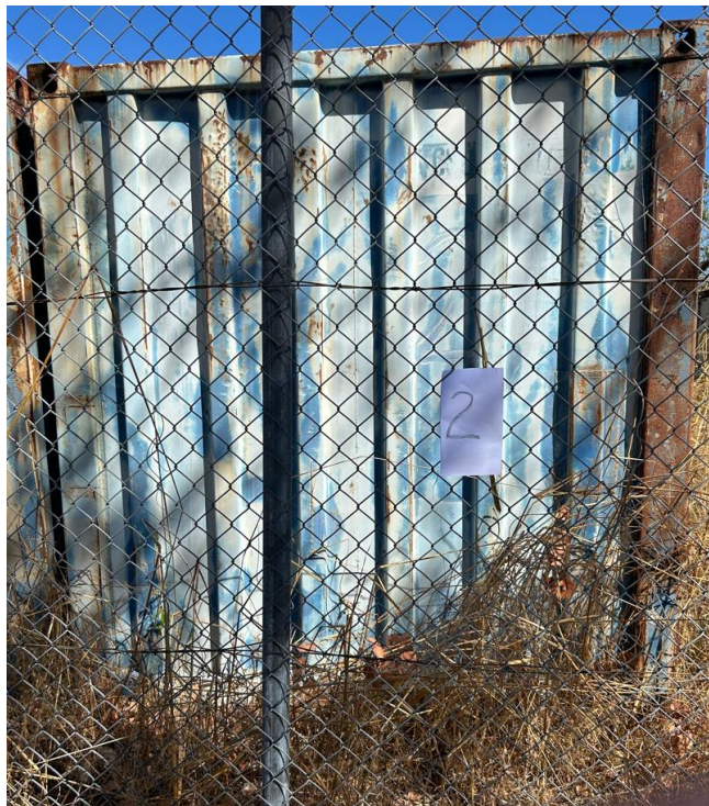
Figure 30. Photo showing condition of end view of shipping container #2
