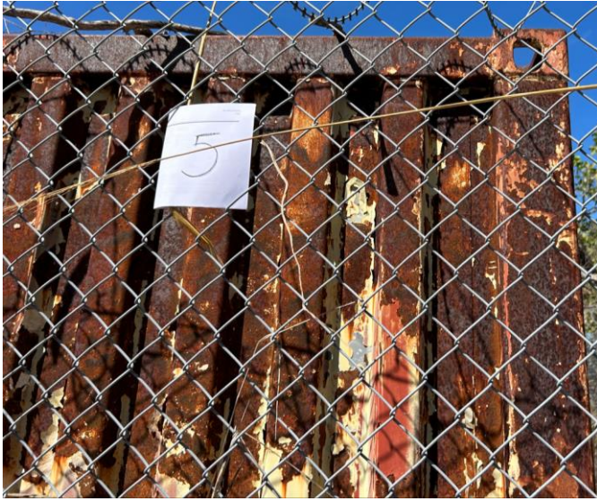
Figure 50a. and b) Close up of the rust on shipping container 5, long fence side, towards the door end, and end side next to shipping container 4
