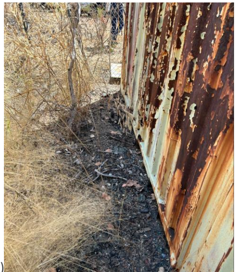
Figure 47a. Buckling of the side wall on container 5, integrity of the container has been breached along the bottom. b) and side c) Close up of rust along the wall looking towards the end of the container.
