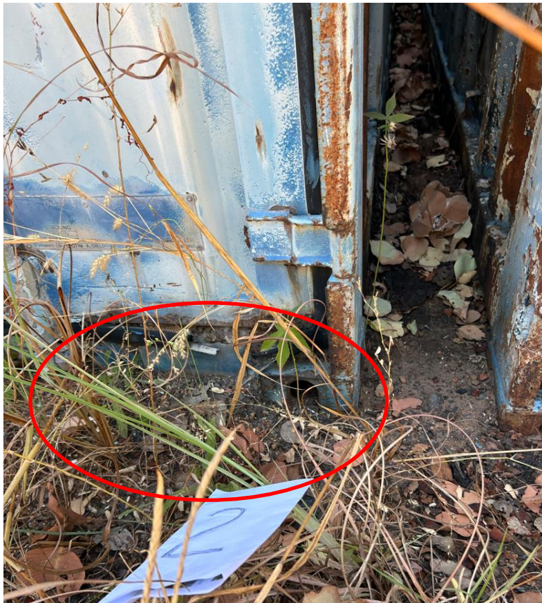
Figure 31. Photo showing some degradation round the bottom door of container 2 and potential sample spill out
