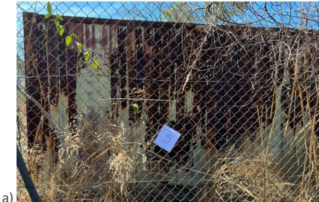
Figure 49a. and b) Photo showing condition of side view of shipping container #5 on the fence side. Rust is clearly visible. The other side of container #5 abuts onto shipping container 4 so no photos of the other long side are possible.
